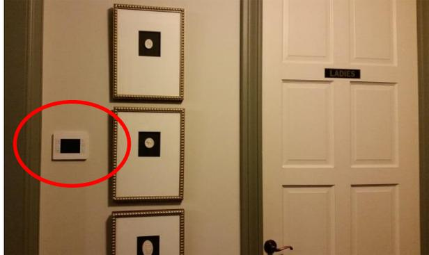
To activate the screen, tap the screen area – the last displayed screen will appear. Press the *main* button to get to the main menu page. If the screen goes blank after a period of non-use, just tap the screen again to reactivate it and the last displayed screen will reappear.
